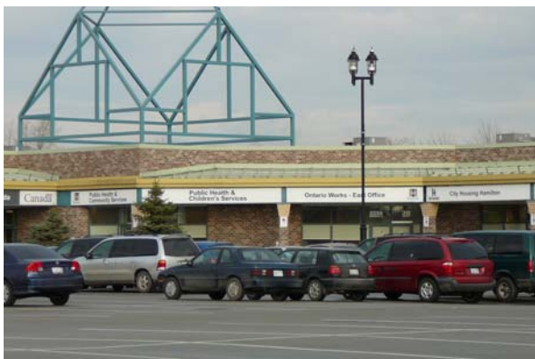
Figure 27: The Public Health office from which the ONF SBS coordinator worked - mall frontage on the outskirts of Hamilton.
