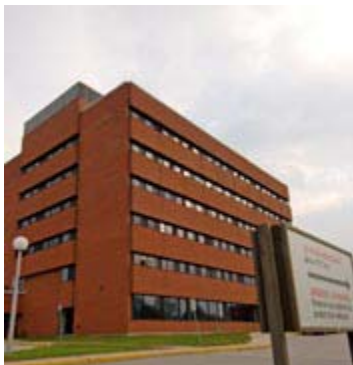
Figure 16: North Bay General Hospital
