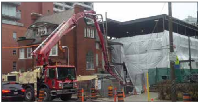
New Spadina Road entrance under construction
